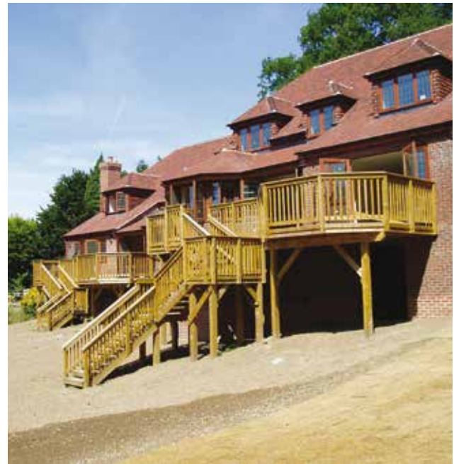
High level decking: Peter Brook Design Ltd.
