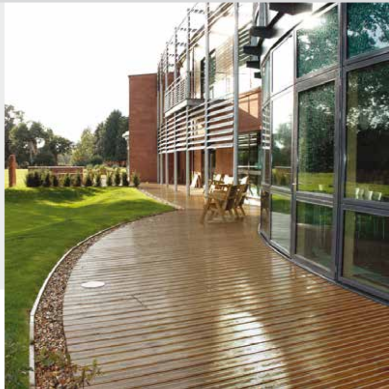
Ground level decking: John Brash & Co Ltd.
